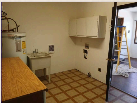
The Laundry Room View
