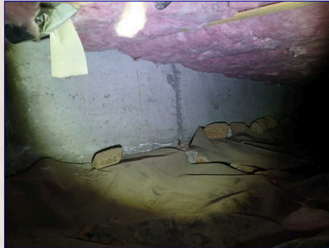
The crawlspace walls view
